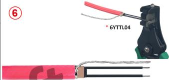
5: Cut and remove the heating section between the two bus wires on the requested length.
