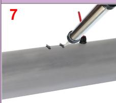
7: Seal the clearance between the metal tabs and the outer sheath of the piping with a silicone or elastomeric sealing resin. Wrap the mechanical protection around the insulation, making two straight cuts for the legs
